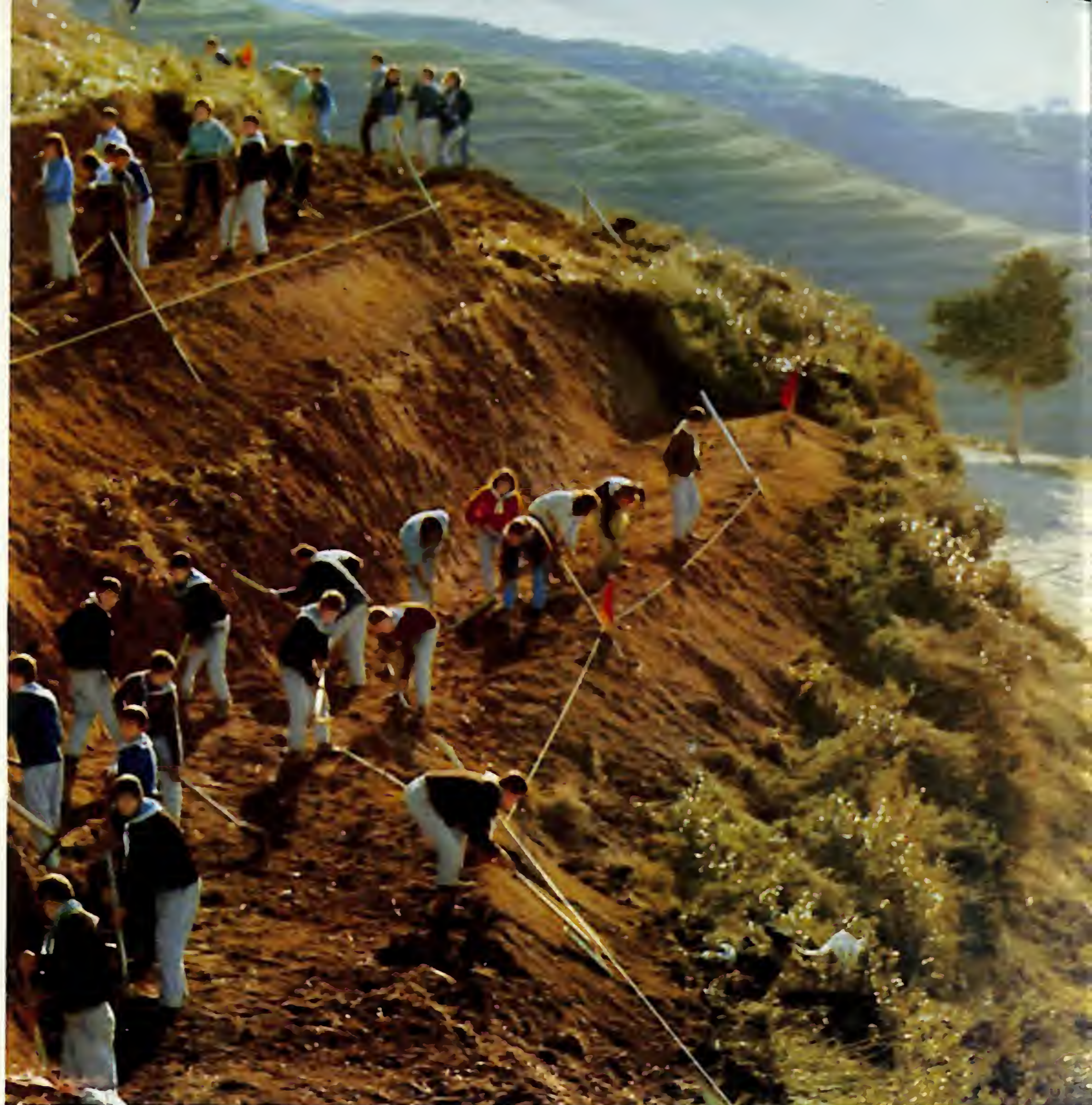
Young volunteer labourers building terraced fields.
